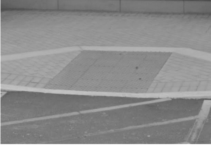
EXISTING ACCESSIBLE RAMP WITH TRUNCATED DOMES
